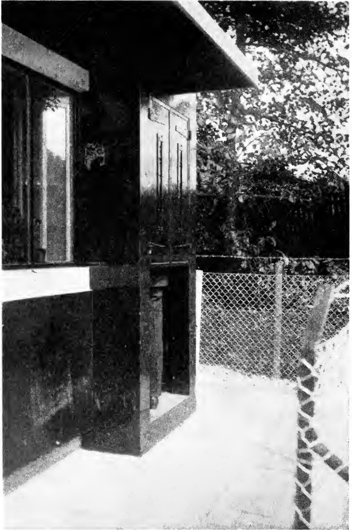
Foreign beat communication equipment: The Hague, Netherlands. Police booth, exterior view, showing how doors only cover upper section (about two-thirds the height of the entrance) so that the lower part remains open and may be inspected from the street.
